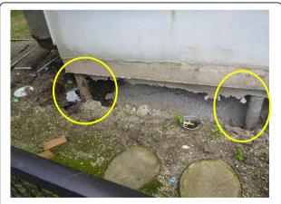
**Fig. 12** The pile foundation of the house which experienced minor inclination in Akitsu
