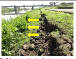
Fig. 10 The occurrence of lateral spreading at the river side, Akitsu
