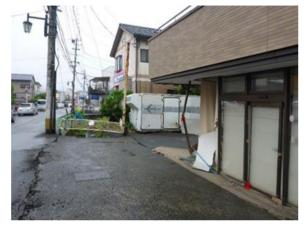
Fig. 3 Example of ground subsidence due to liquefaction
