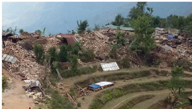
**Fig. 13** Completely collapsed dry stone masonry houses in entire neighborhood of western Nepal after 2015 Gorkha earthquake
