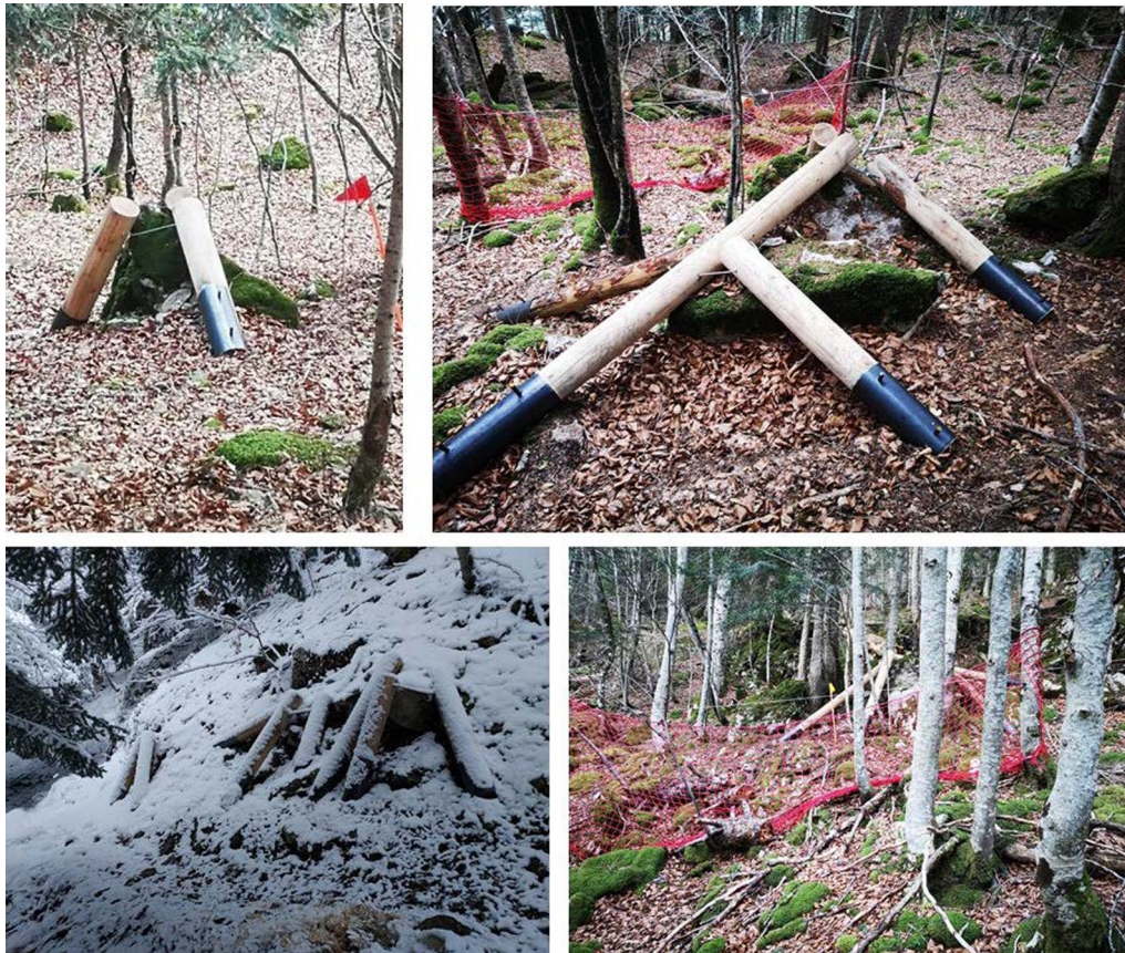
Fig. 9 Examples of implemented protective structures in the slope at Artouste (Photo: S. Fábregas)
