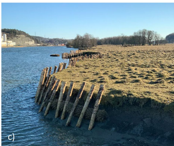
Fig. 12 Three testing areas along the Göta river (Sweden) where different NbS for riverbank erosion due to ship waves are implemented: a wooden pier filled with Christmas trees; b submerged stone barrier; c coir logs fixed with wooden piles. (Illustrations P. Danielsson, SGI)
