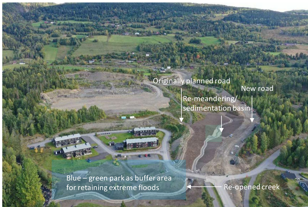
Fig. 11 Drone photos of the Trodalen site in Øyer municipality, Norway, after completion of the interventions, but before planting along the streambanks is fully completed (Solheim et al., 2023)
