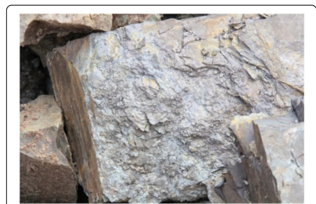
Fig. 9 Photograph of the silty mudstone of the potential slide surface
