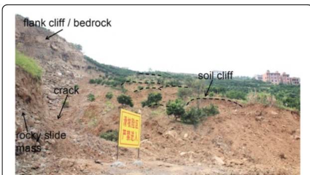
Fig. 8 Photograph of the crack trough between the rocky slide mass and the northern slide mass, and the soil slide cliff created by the soil mass slide
