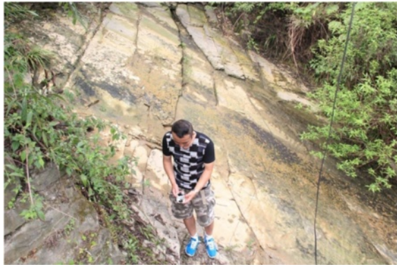
Fig. 10 Weathered surface of the preexisting sandstone layer, 20 m from the northern boundary of the landslide
