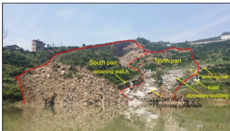
Fig. 5 Panoramic view of the Shanshucao slope after failure (taken on Sept. 4). No remnants of the hydropower station can be seen in the ruins
