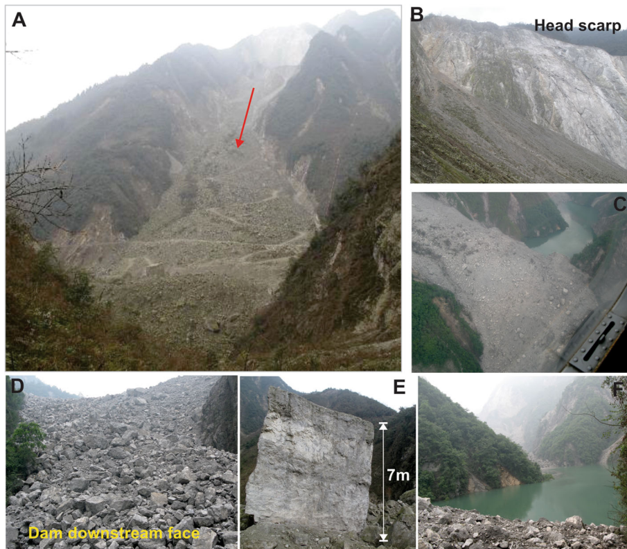
Fig. 5 Laoyingyan landslide. a Overview of the Laoyingyan landslide; b Head scarp; c Helicopter view of the dam body; d Dam downstream face; e : The largest boulder in the deposition zone; and f Barrier lake
