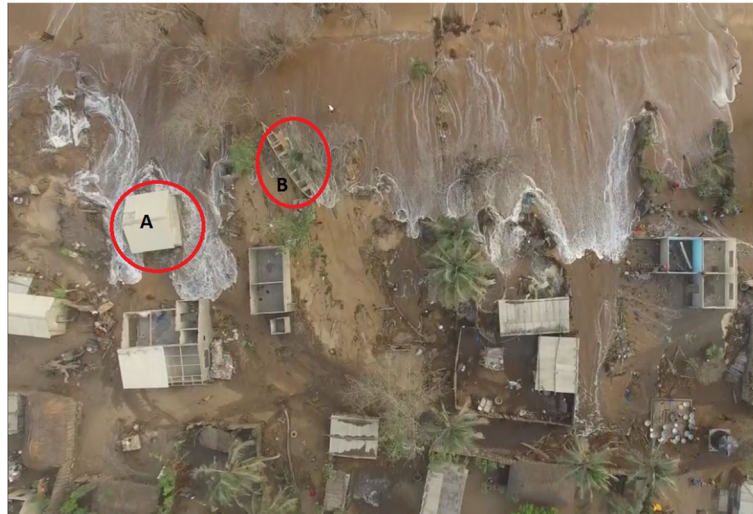
Fig. 9 Flooding in Fuvemeh affecting buildings (A) and fishing canoe (B)
