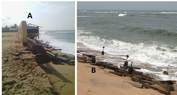
Fig. 7 State of the school building in May 2016 (a) and June 2016 (b)
