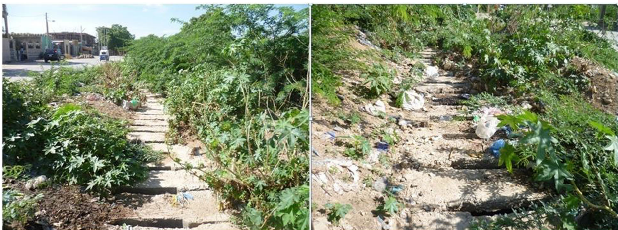
Fig. 7 Vegetated drainage line at Gate no.2 of Dire Dawa University
