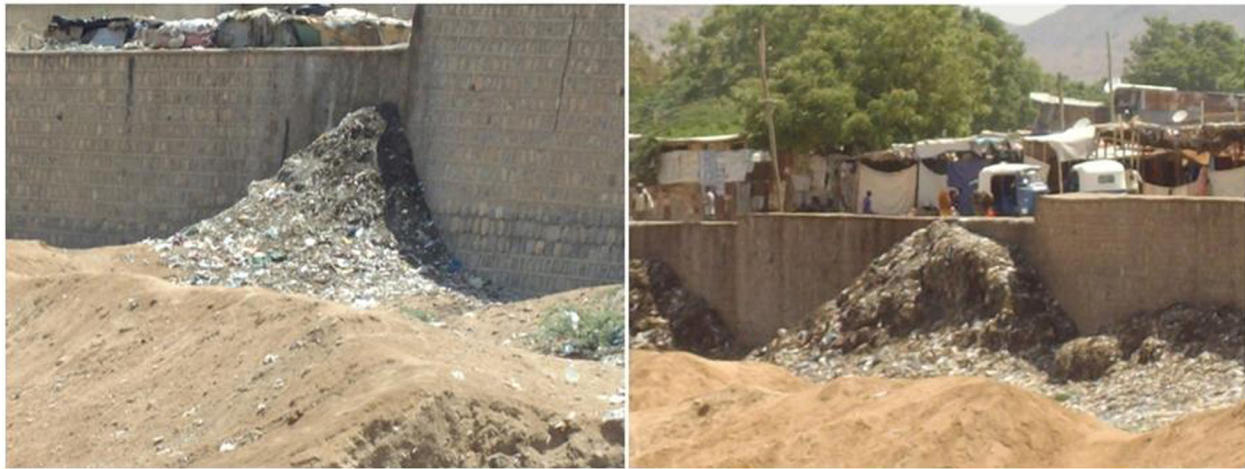
Fig. 6 Solid waste dumped into Dechatu River across the flood protection wall
